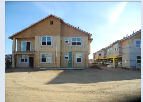
Photo of construction of Sierra Village Project
